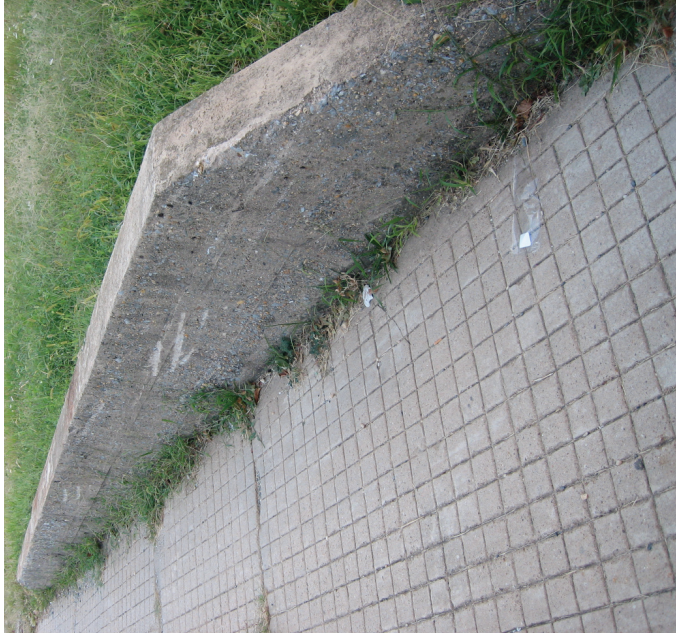
Recycling sources: Site walls and driveways
